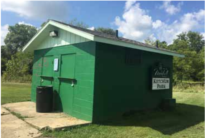
UPPER PARK RESTROOM (CLOSED)
