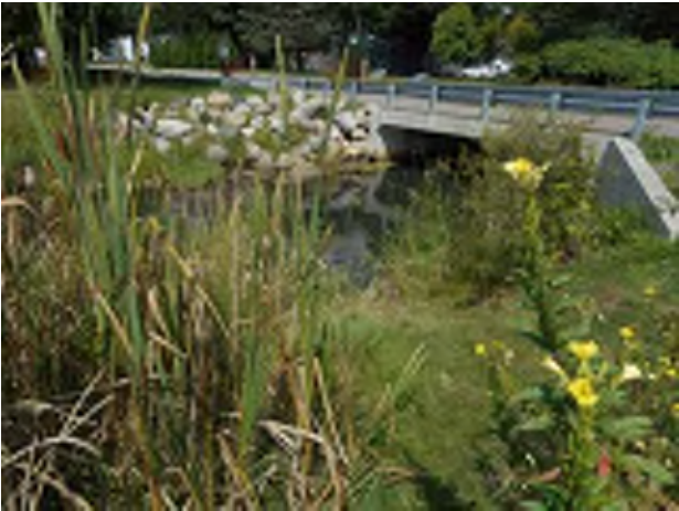
NORTH ENTRANCE VEHICULAR BRIDGE
