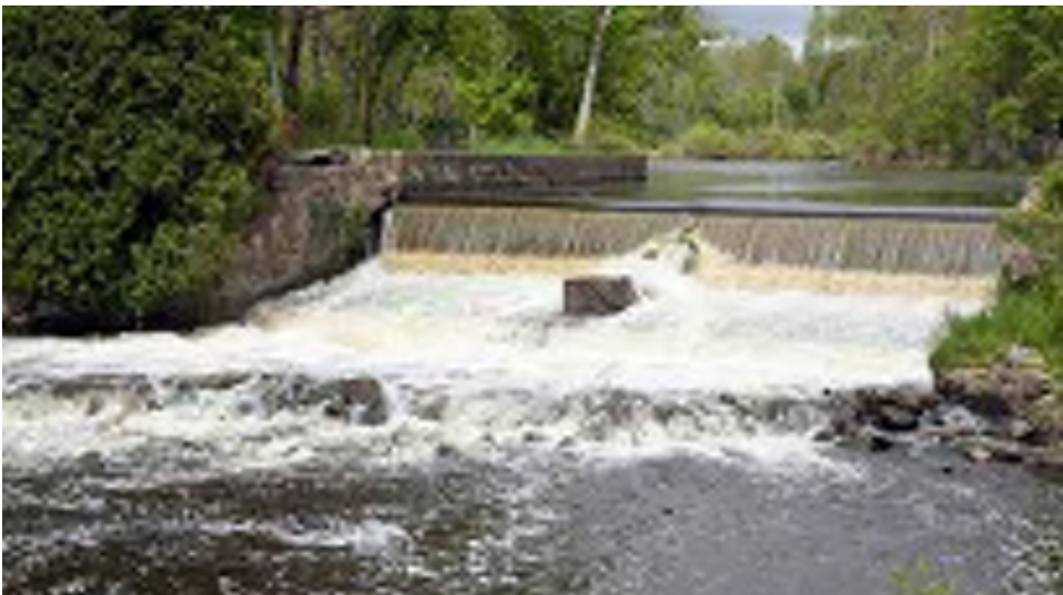
FORMER SPILLWAY AT WEST END OF PARK
