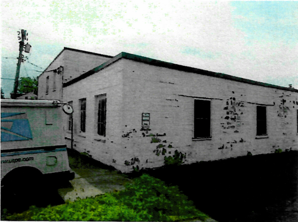
View of the northwest corner.
