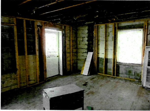
View of upper level.
