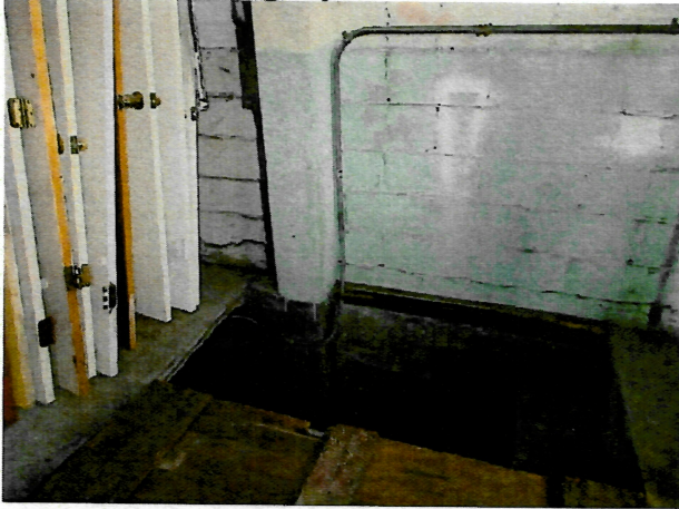
View of basement entry.
