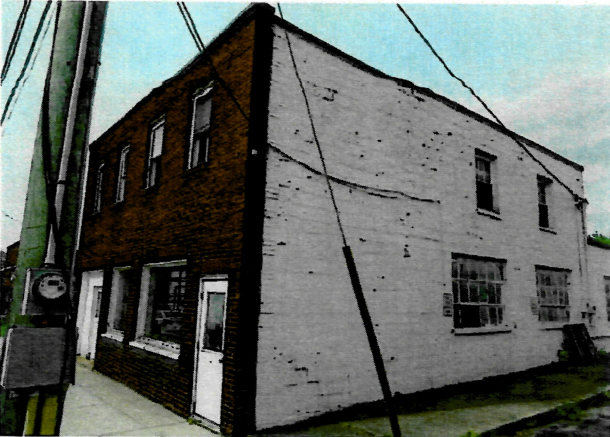
View of northeast corner.
