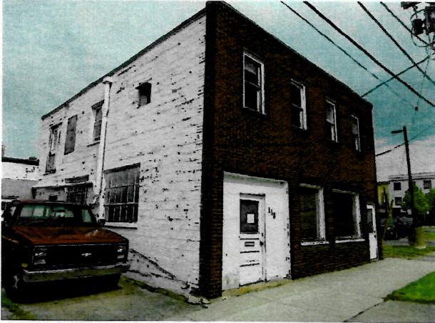
View of the southeast corner.
