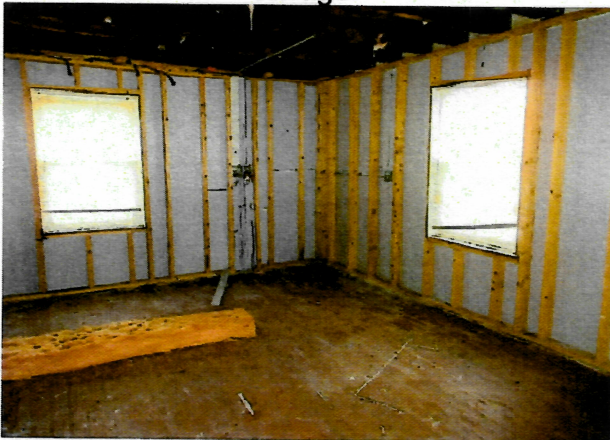
View of upper level.
