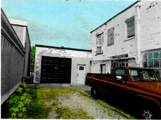
View of the south side.
