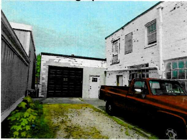
View of the south side.
