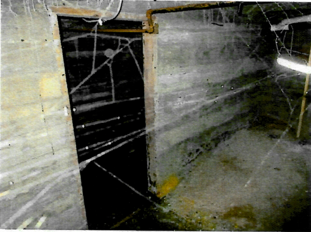
View of basement storage.
