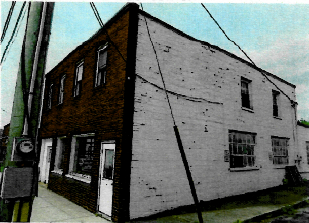
View of northeast corner.
