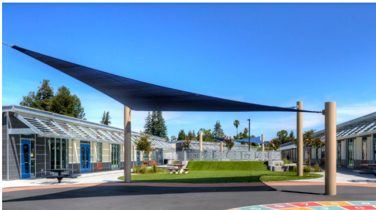
Shade sail design working off of existing light poles
